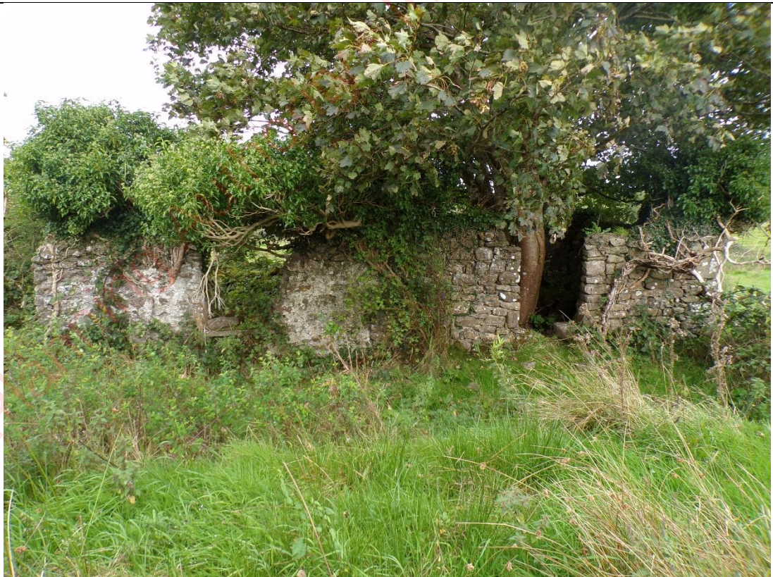
Plate 14-4: Vernacular building CH29, facing west.
