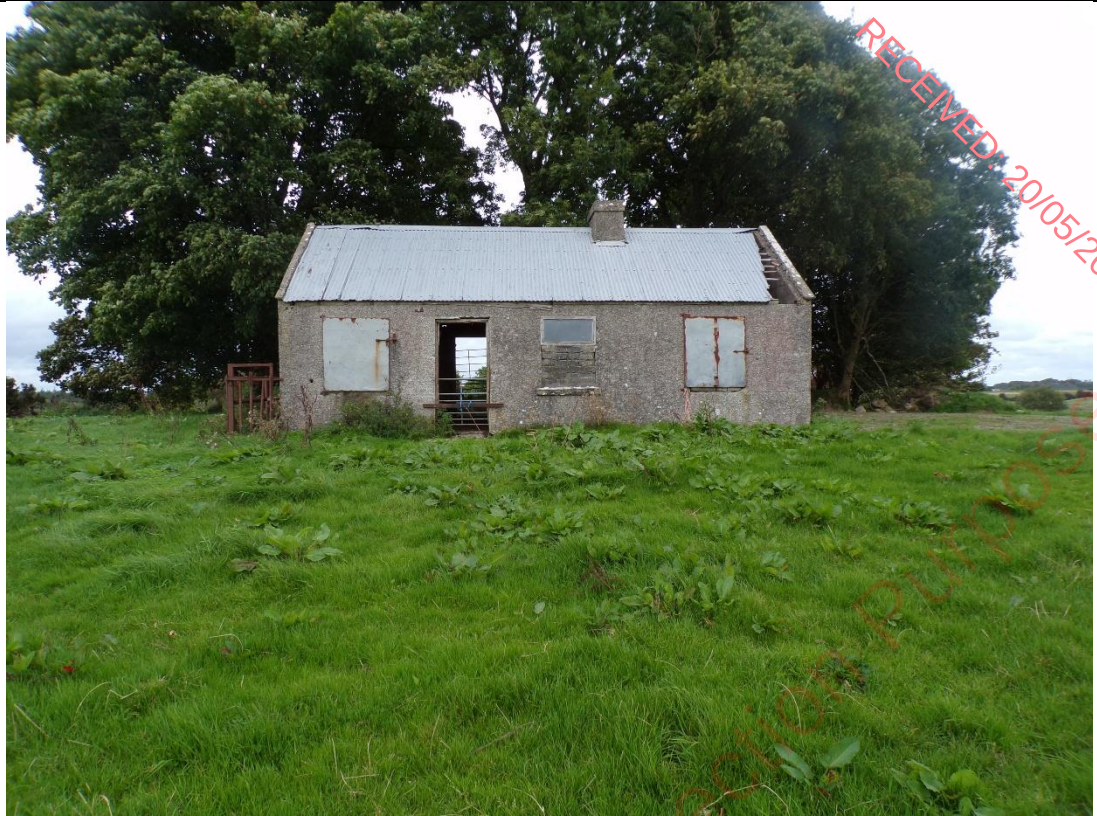
Plate 14-5: Vernacular building CH46, facing north.
